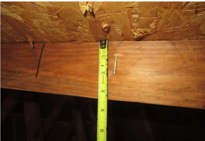
8d nails verified
