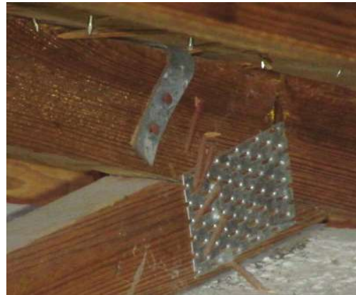
Single wrap with at least 2 nails on the embedded side and at least 1 nail on The wrapped side
