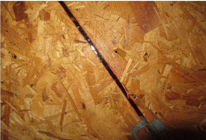
SWR installed under the shingles
